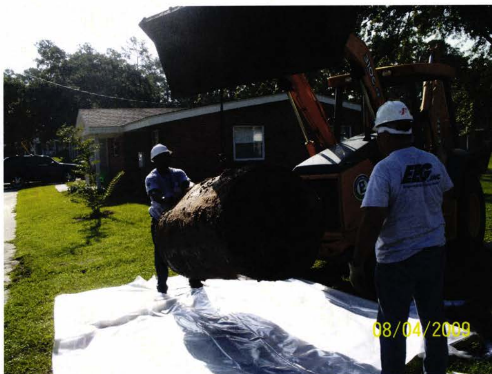
Picture 2: UST 1447Dove.
